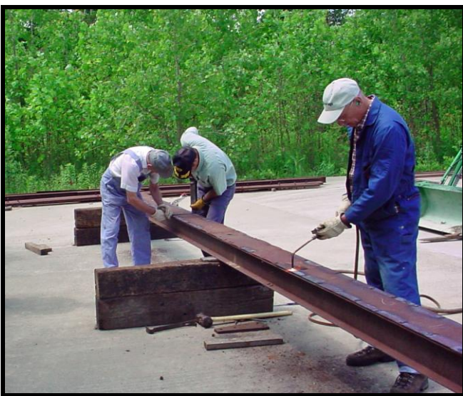
Removing pack rust from a Stearns truss bridge in Delphi Indiana
